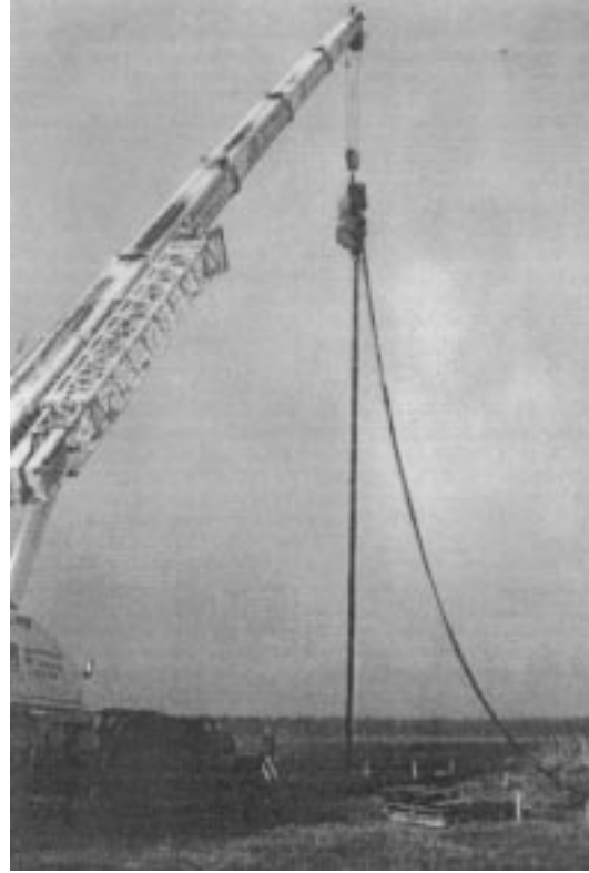
Figure 6. Pneumatic-dynamic sound with airgun before lowering.
